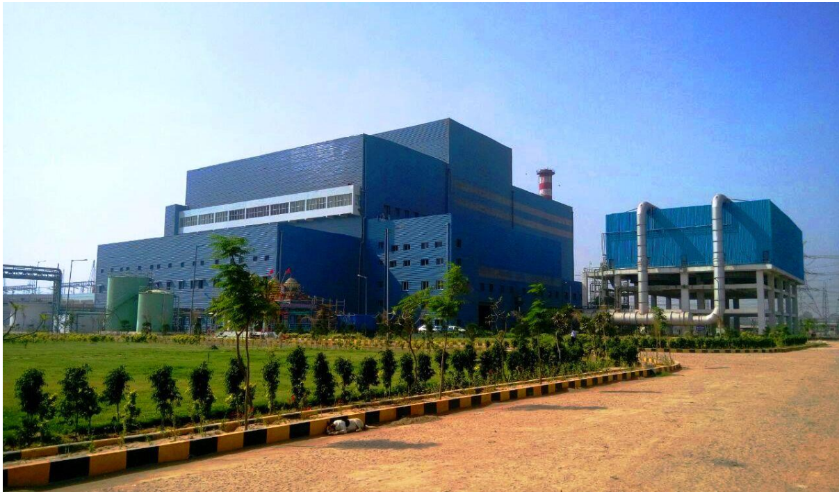
2 x 600 TPD MSW Based Power Plant in Delhi
